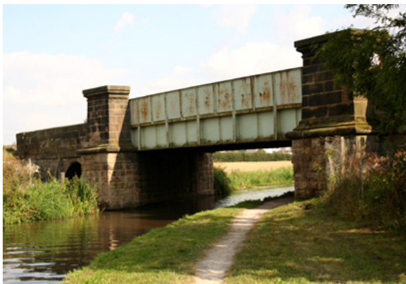
Below - railway bridges over the canal. Left; bridge near Stenson Junction incorporates giant stone piers with rusticated stone bases & cornices & riveted iron plate box-girder construction. Right; smaller scale bridge of similar construction at Weston Lock, with handrail to parapet
