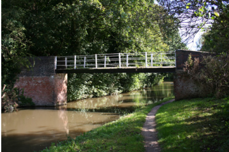
Above left & right - pedestrian footbridges over the canal. Bridge No. 10 at Cliff Wood (left) was always a narrow footbridge, which catered for packhorse traffic approaching the river crossing. The cast iron posts & wrought iron rails are 20th century & probably replaced a timber fence. The footbridge at Weston Lock (right) has a cast metal deck & is a pattern repeated at the locks.
