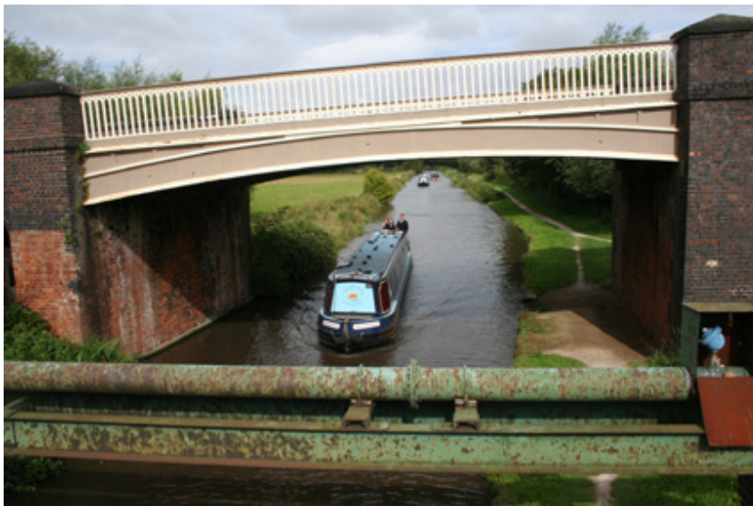
Below - railway bridges over the canal. Left; bridge near Stenson Junction incorporates giant stone piers with rusticated stone bases & cornices & riveted iron plate box-girder construction. Right; smaller scale bridge of similar construction at Weston Lock, with handrail to parapet
