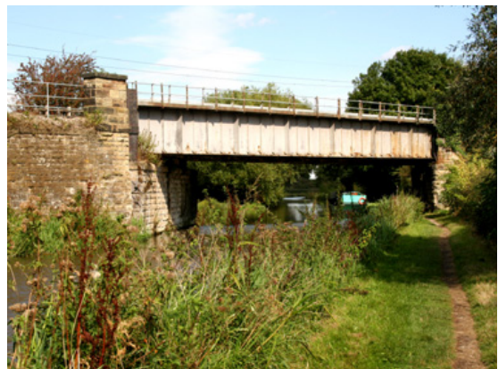
Below - railway bridges over the canal. Left; bridge near Stenson Junction incorporates giant stone piers with rusticated stone bases & cornices & riveted iron plate box-girder construction. Right; smaller scale bridge of similar construction at Weston Lock, with handrail to parapet
