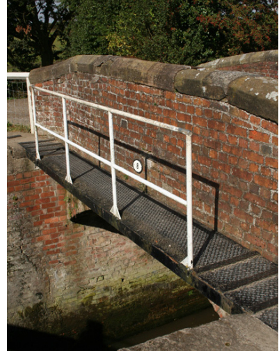
Above left & right - pedestrian footbridges over the canal. Bridge No. 10 at Cliff Wood (left) was always a narrow footbridge, which catered for packhorse traffic approaching the river crossing. The cast iron posts & wrought iron rails are 20th century & probably replaced a timber fence. The footbridge at Weston Lock (right) has a cast metal deck & is a pattern repeated at the locks.
